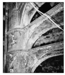
Lead paint must be removed from the spiral staircase before repainting, but the cast-iron is solid.
