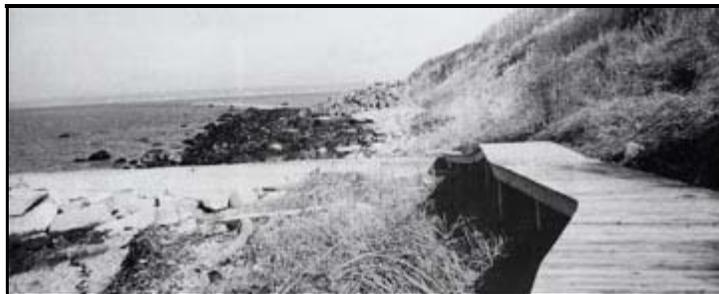
A new walkway, completed in November, now connects the concrete jetty to the boathouse. A new floating dock is planned. Visitors will debark on the floating dock, then walk up a ramp to the concrete jetty and follow the new walk to the boathouse. Built by Roland Greenvall of Stony Creek, the new walk required seven days of work by a crew of three. The crew stayed overnight in the generator building during construction. Photo by Fred Farnsworth.
